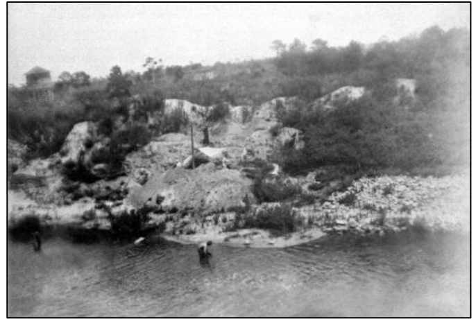
"View of canal showing where excavation for human remains was made" Image from State Archives of Florida, Florida Memory.
