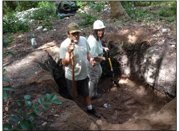
Bob and Chris leveling and tamping the fill as it is being deposited into the unit.
